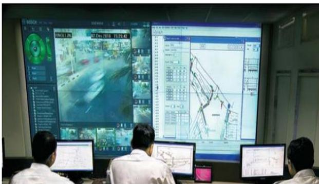
The traffic in Mumbai is dynamic. Instead of using pre-defined algorithms based on theoretical traffic volumes, the adaptive signalling system that operates in Mumbai collects various real time parameters such as traffic flow, traffic intensities, traffic queuing and vehicle waiting times at traffic intersections and relays this to the Area Traffic Control Centre. This information is used to dynamically adjust offsets and calibrate signal timings to accommodate changing traffic conditions.
